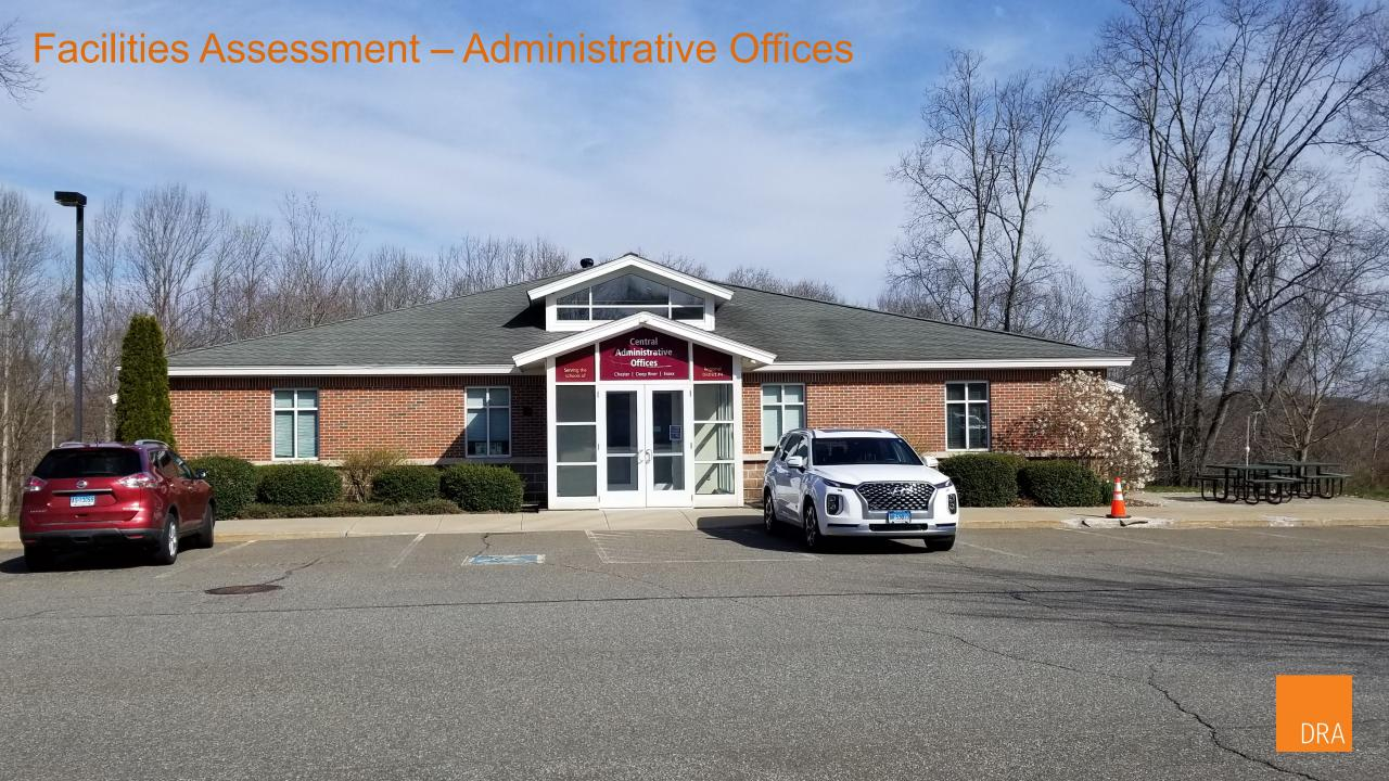
Roof at ~50% life remaining Mortar deterioration Staining to walls Not ADA compliant Deteriorated walkways Crosswalk not compliant
